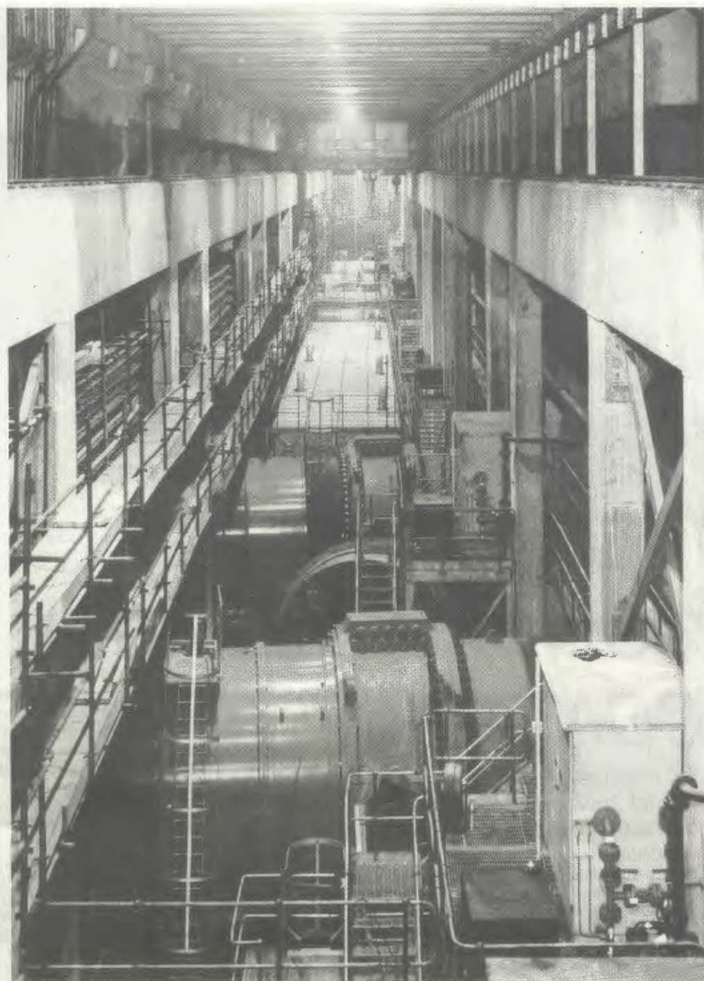
Just one of the giant holes scooped out of the Power Mountain. Nearly 200 yards long, 25 feet wide and about 65 feet high, this cavern houses the enormous draft tube valves which serve as isolation valves for the lower lake.
